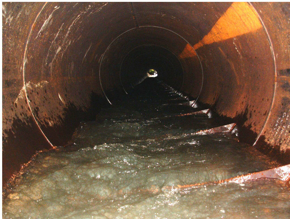
Figure 8.15 Baffles slowing water velocities at high flows while producing minimal turbulence, John Hatt Creek
