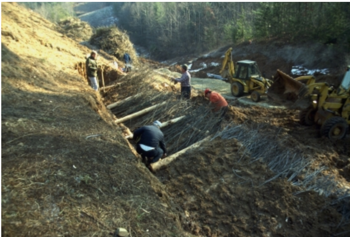
Figure 18-17 A live cribwall being installed (Robbin B. Sotir & Associates photo)
