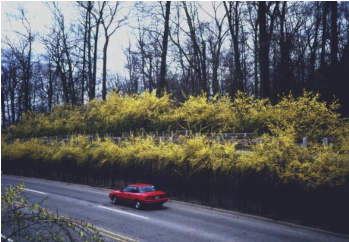
Figure 18–27 A tiered wall with bench plantings (Donald H. Gray photo)
